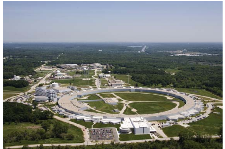
Aerial view of the Advanced Photon Source.
